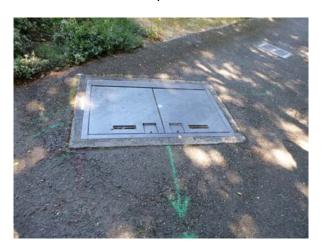
**Flow Meter Vault:** A new flow meter will be installed in line with the existing 4-inch forcemain along the westside of 116th Place SE. The flow meter will be installed within a new 4-foot by 4-foot precast concrete vault with a H30 traffic rated lid.
